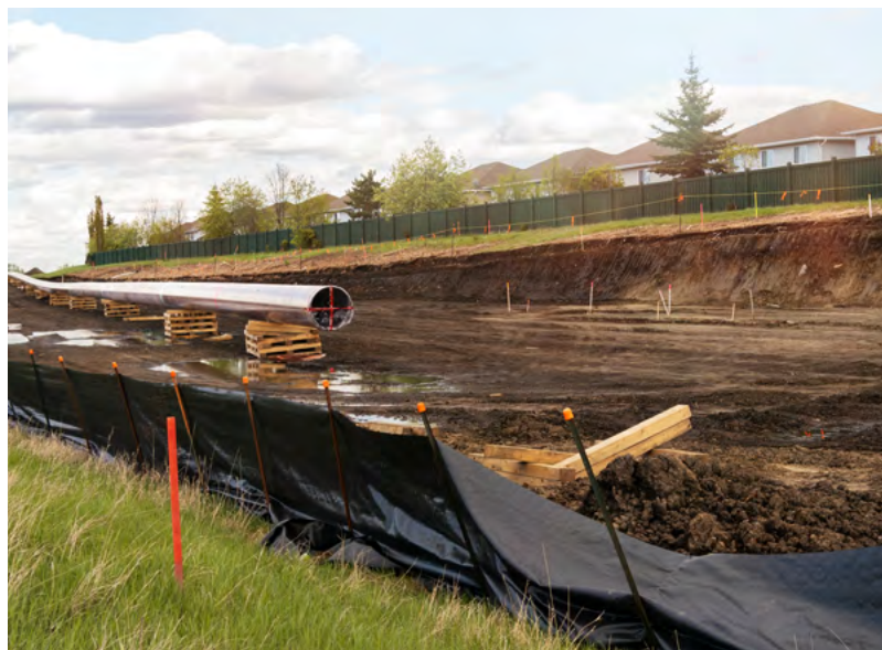
Construction of Trans Mountain Pipeline in Edmonton, Alberta. (Photo: iStock)
